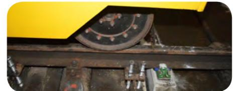
*Example of a track rehabilitation with Corkelast® EBS RF installed in between daily operations*
