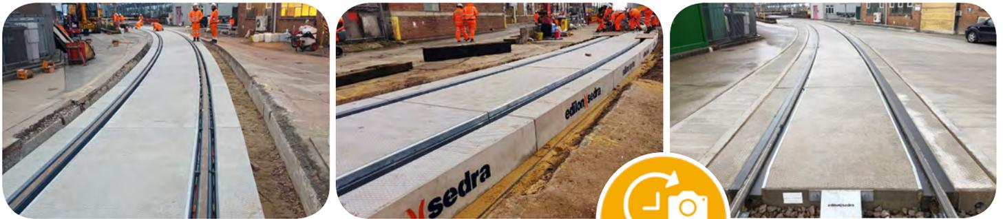
Installation of Corkelast® LCS-350 in the Ruislip Depot, for London Underground
