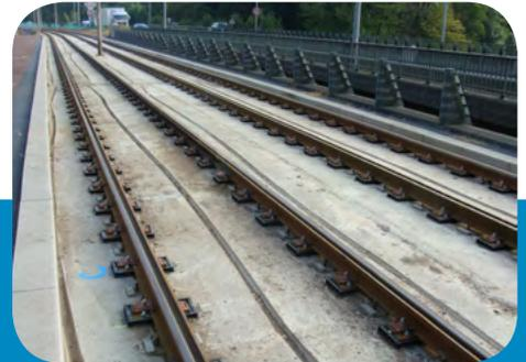
*Installed new baseplates and application with Dex<sup>®</sup>-G for tramway Orléans*
