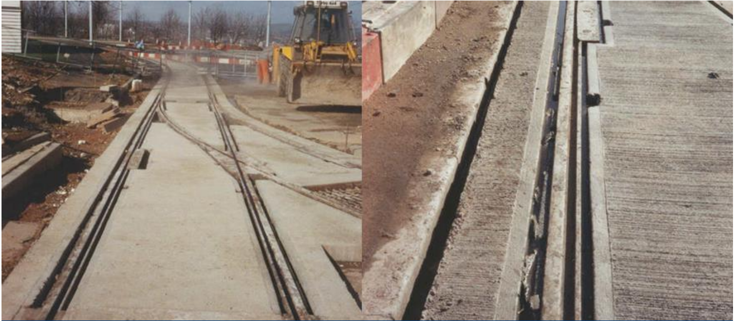
Construction of the concrete slab track
