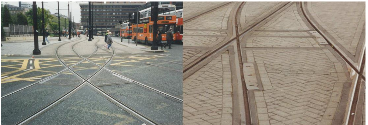
edilon)(sedra Corkelast® ERS (Embedded Rail System) in combination with asphalt and stone paving
