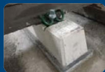
Apply fast curing grout
