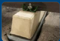
Fix EBS-RF block unit to rail
