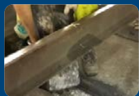
Remove old sleeper from recess
